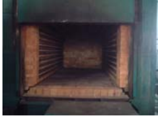
Furnace for Heat Treatment
